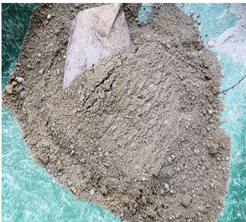
Fig 1 Mixing of mortar for ECC Concrete
