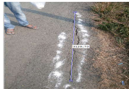
Figure 5 Longitudinal cracking
