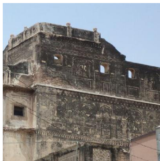
Figure1 Desert Varnish growing on an ancient building located at Bikaner city of Rajasthan
