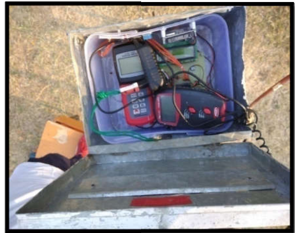
Fig 2 Module of weather monitoring system
