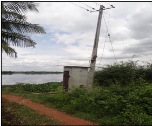
Figure 20& 21 Constructed huts and ground water pump house at shores of reservoir.
