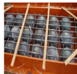
Hollow elliptical balls
