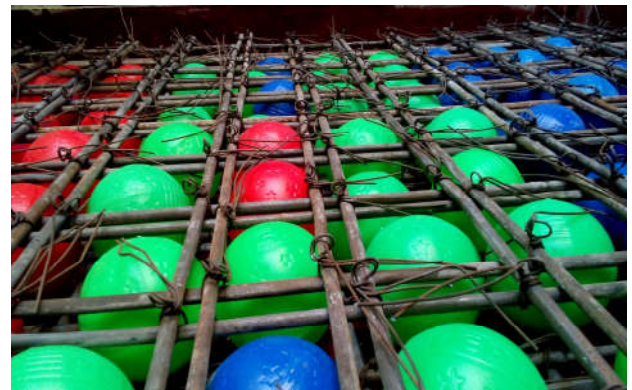
Fig 5 Reinforcement of continuous bubble deck slab
