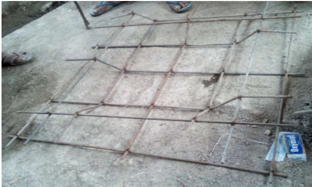
Fig 2 Reinforcement of conventional slab
