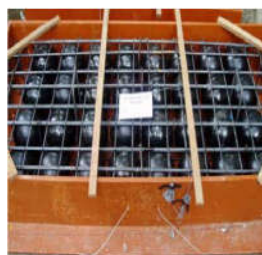
Hollow spherical balls
