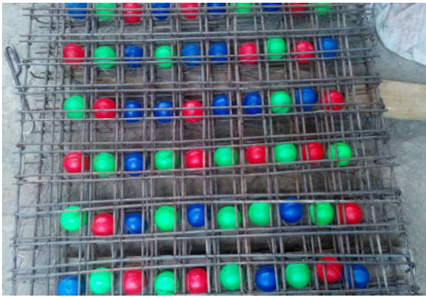
Fig 7 Reinforcement of Alternative bubble deck slab (type II)
