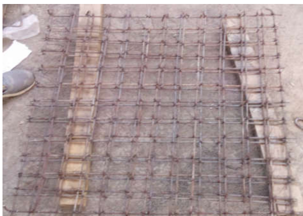
Fig 3 Reinforcement of bubble deck slab
