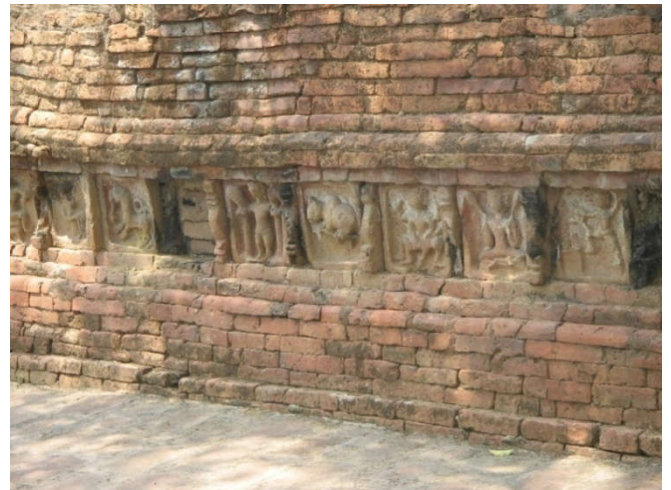
The plinth of a brick temple
