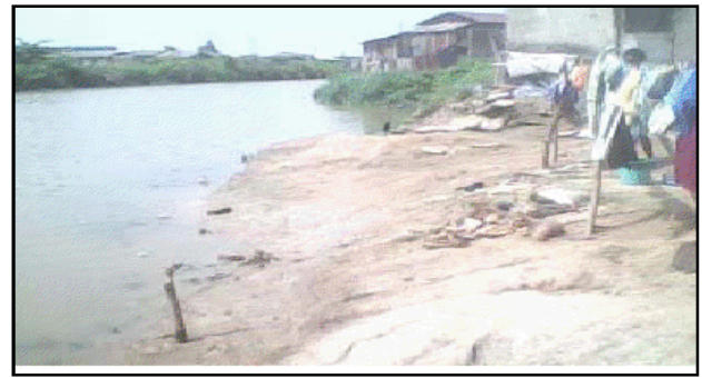
Figure 6 Building constructed along flood plain in the NDR
