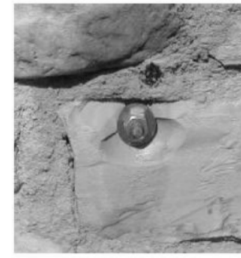
(a) by injection (b) transverse bars fixed with bolts
